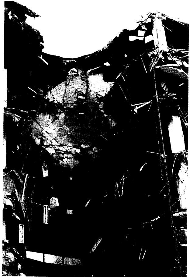
The "Mother Slab" or "Slab from Hell" hangs by a few strands of steel rebar at the top of the "Bowl." Estimated to weigh 35,000 pounds, it caused concern for several days until it was finally anchored to the rear of the structure.
