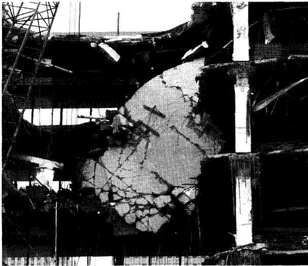
"Mother" hangs from the top floors of the Murrah Building after being pinned and strapped to the south wall. Snow fencing is placed to prevent debris from falling from the upper floors.
