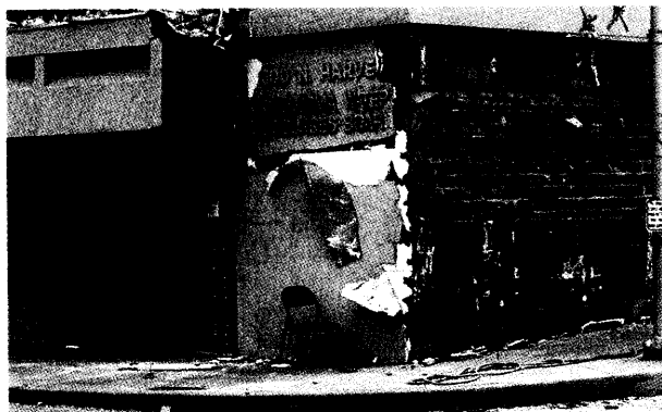
The Oklahoma Water Resources Board Building shows the scars it received from the massive explosion across the street. The Murrah Building was not the only structure that suffered damage, and federal employees were not the only people injured or killed.
