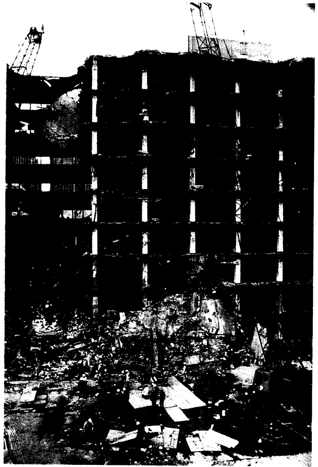
After removing tons of "widow makers" and installing snow fencing on upper floors, crews prepare for their final assault on the "Pile" and "Bowl" areas.
