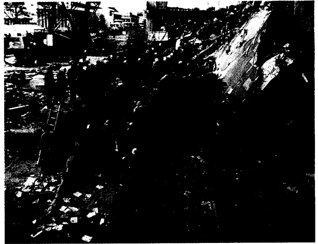
Personnel from various agencies work on the north debris piles from the "Bless Slab" (foreground) to the east wall of the Murrah Building.
