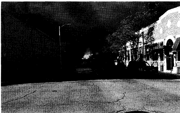
Smoke from approximately 40 car fires ignited by an explosion billows skyward, obscuring the view of the main target of the terrorist attack. A one-story addition to the Journal Record Building (left foreground) has suffered extensive damage. A brick office building (right) has also been heavily damaged.
